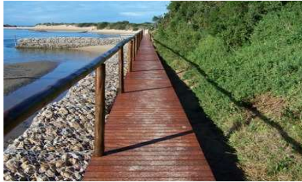
New wooden Walkway
